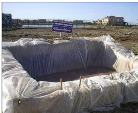
Plate 3-1 Typical concrete wash out areas
